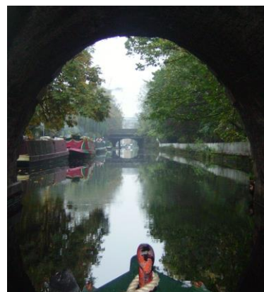
Islington Tunnel still standing
